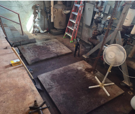
Boiler pieces outside in the parking lot
