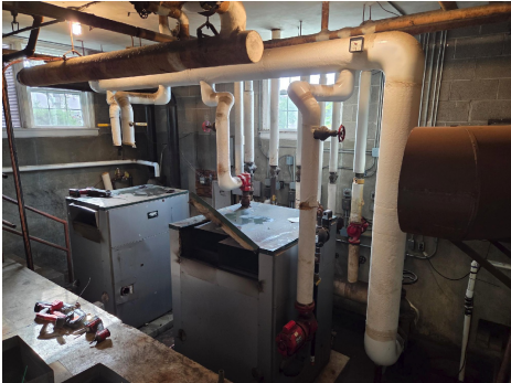
Wide angle of Boiler Room
